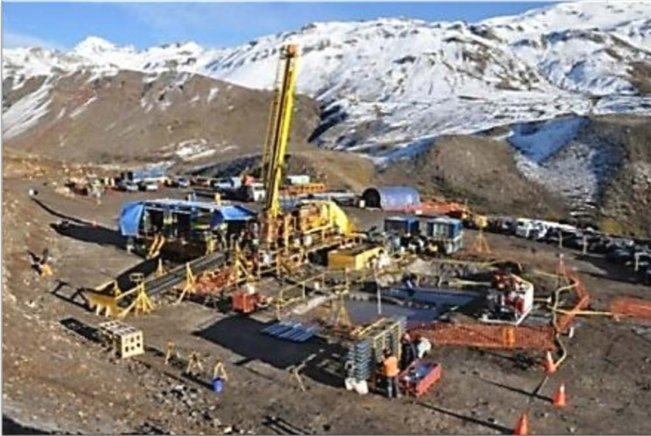
Alterra power, Mariposa geothermal project, diamond drilling 3 well campaign.
