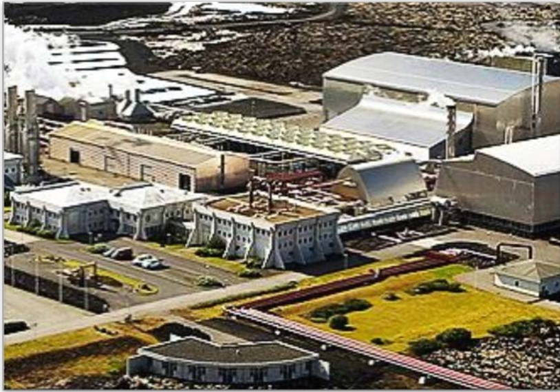
HS Orka, Svartsengi, Iceland 75 MWe geothermal power plant
