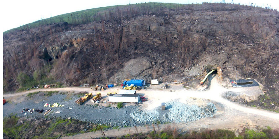
Aerial View QWest - A Zone Portal
